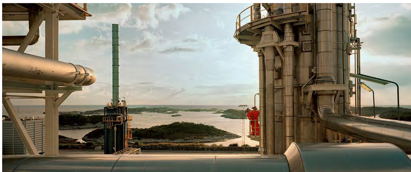
Kollsnes gas processing plant at Øygarden, Norway.
